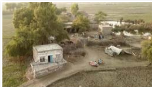
Building nine houses in flood affected village (Noor Muhammad Kashkeli).
