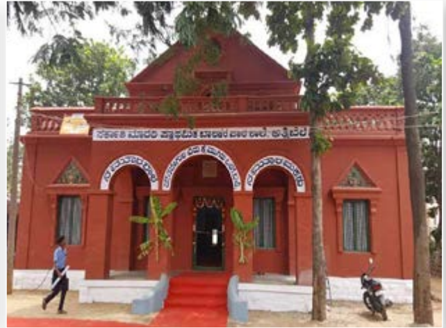
Restoration of a heritage building of a government school (2016).
