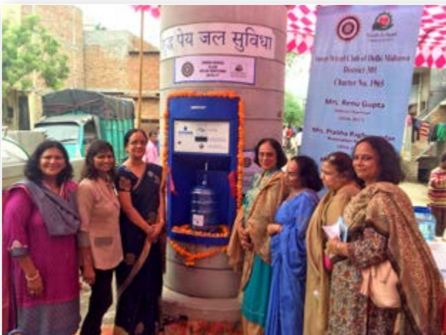
Installation of a potable water kiosk.
