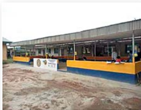
Shelter built and donated by the Inner Wheel Club of Ikorodu Metropolitan, District 912, at the primary health centre for pregnant and nursing mothers, commissioned on 25 Jun 2021.
