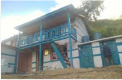
Community house built for villagers in the very far west of Karanga village in Nepal.
