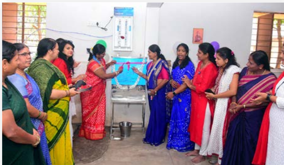
Installation of a reverse osmosis water plant in a school.
